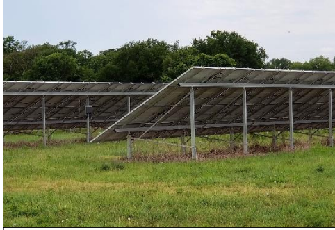
Example of a Solar Conversion System, Ground-mounted
